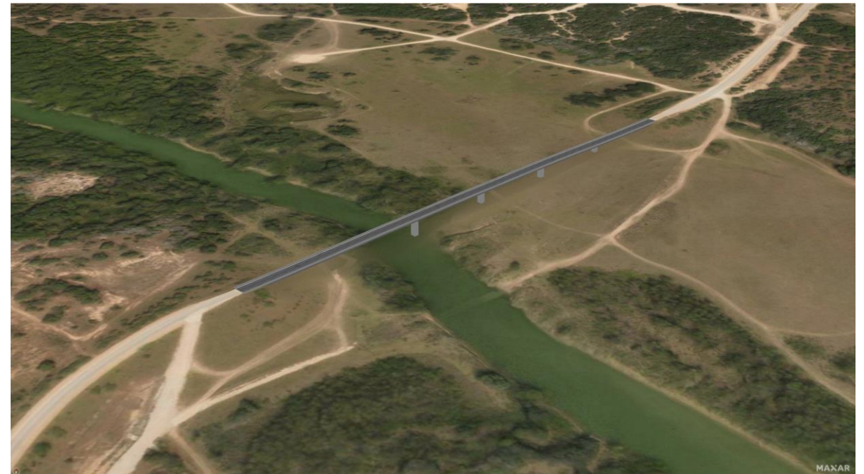
Imagery Under Bridge Procedurally Painted Out
